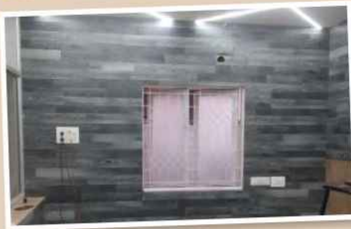
Flooring used in Wall Paneling
