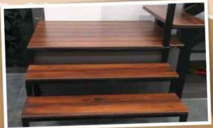
Flooring used in stair case
